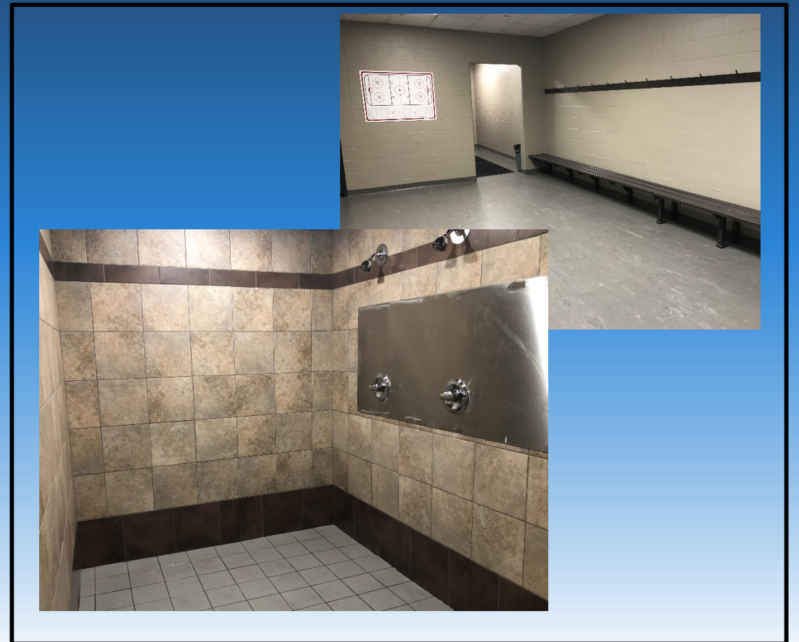
Long Sault Arena Renovations to the Changerooms & Canteen
