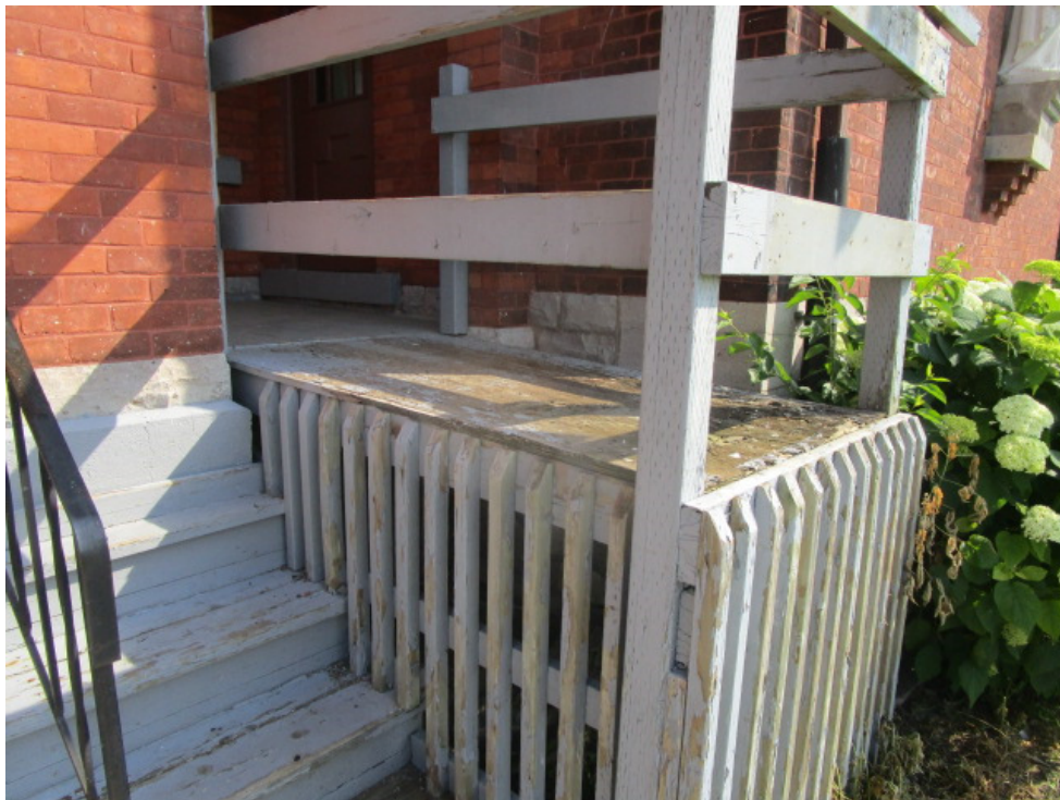
Photo 22 – Front Entrance Landing And Stair Condition
