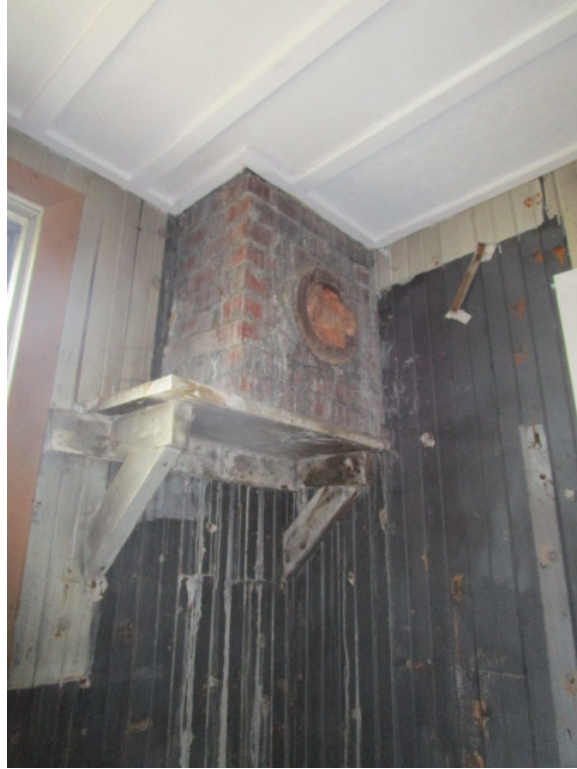
Photo 21 – Chimney Structural Support
